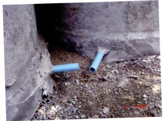
Figure 2 Drainage holes at the bottom of the containers
