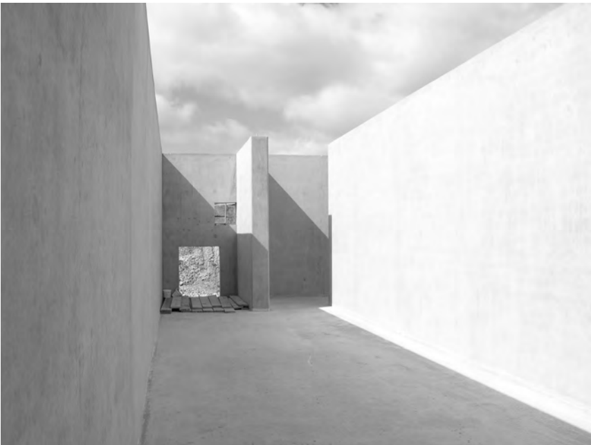
Figure 1.2 A concrete tank (before construction of the roof) illustrating the simplicity of the structural form (Photo: M.J. Kirby).
